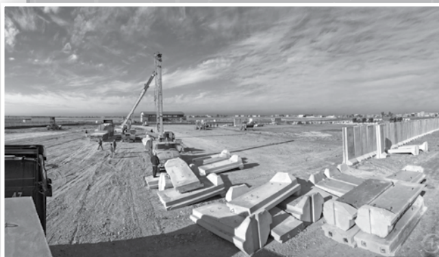
Construction of hospital's blast walls, Bartella
